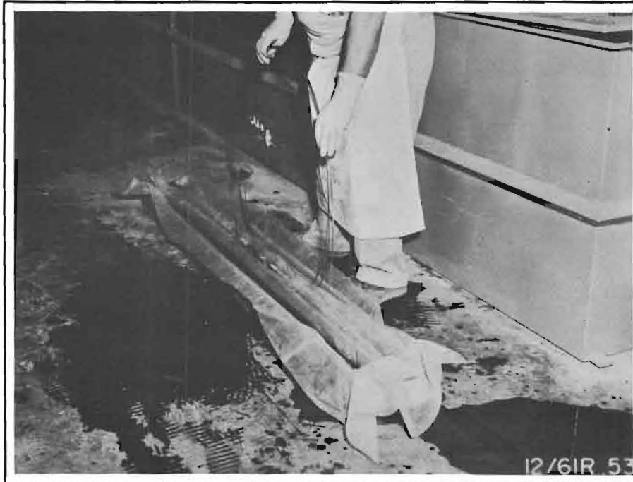
Figure 13. Dipping stressing wires in dilute hydrochloric acid to etch the surface of the wire and improve the bond between the wire and the concrete.
