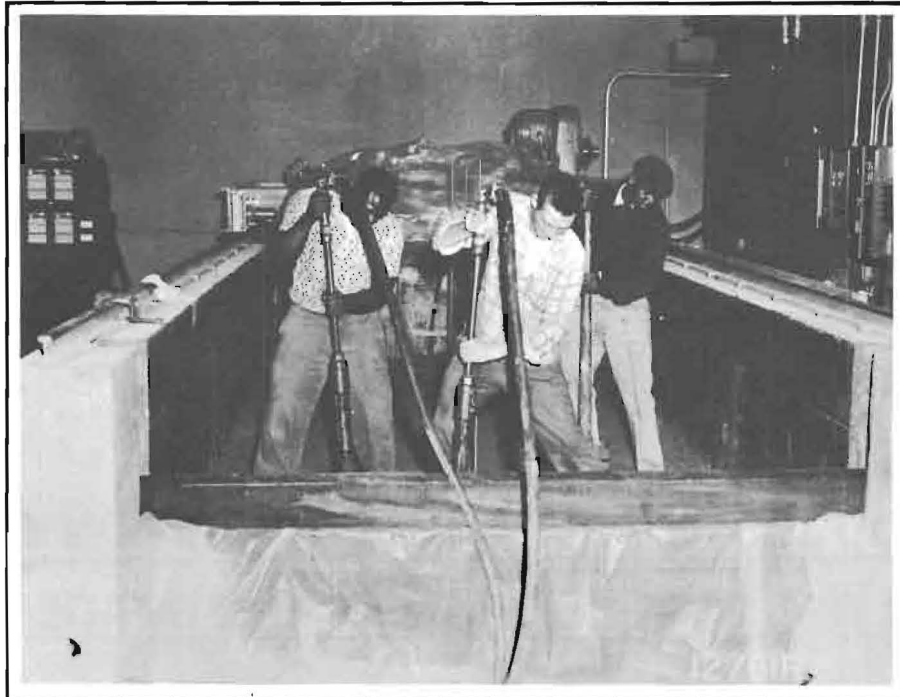
Figure 8. Compaction of the clay subgrade using pneumatic tampers.
