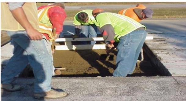
**Figure 5.** Initial cleaning and preparation of the base.
