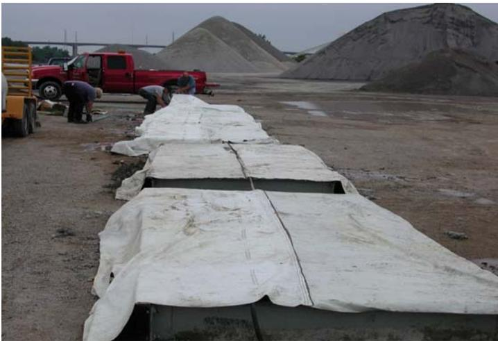
d) Curing of precast slabs.
