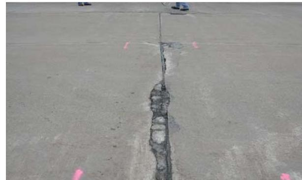
d) Deteriorated joint with spalling.
