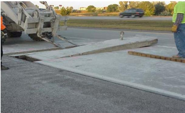
c) Removing the existing slab.
