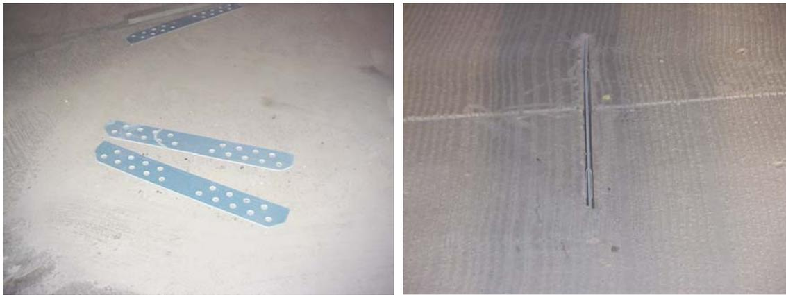
**Figure 25.** Fiberglass stitches.
