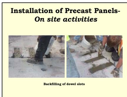
Once the slab elevations are verified and deemed acceptable, the dowel slots are grouted and the joints are sealed.
