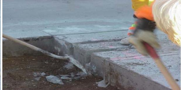
b) Debris removal from dowel slots.
