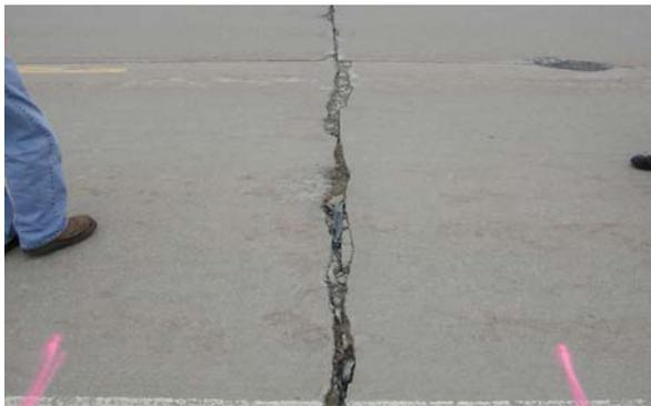
c) High-severity transverse crack.
