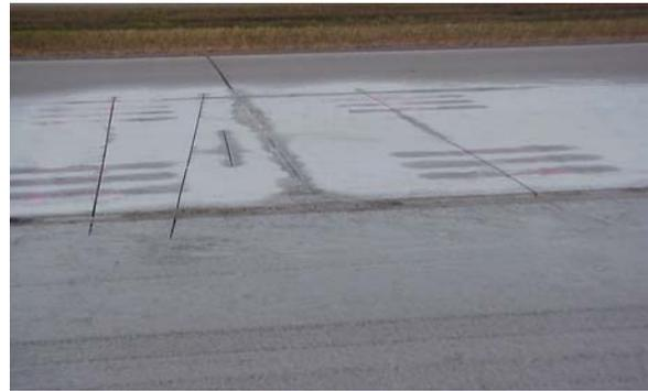
b) The existing slab after sawcutting.
