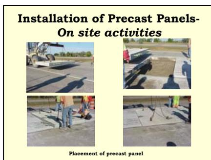
The precast panels are transported from the flat-bed truck to the excavation using a front-end loader.
