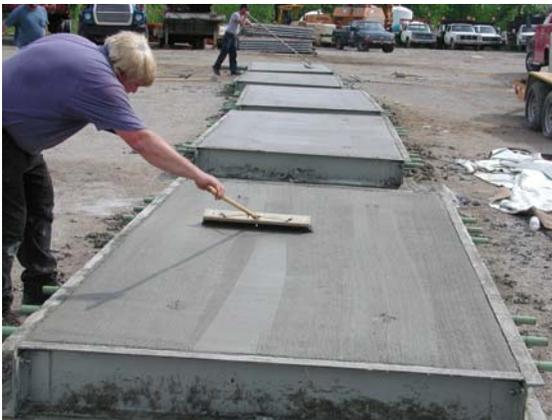
b) Concrete placement for precast panels.
