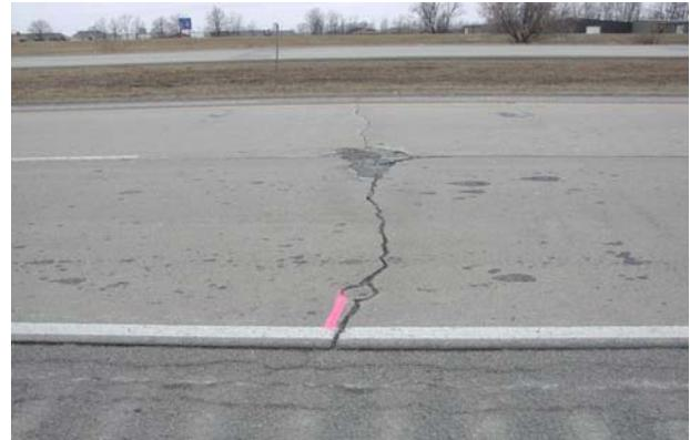
b) Medium-severity transverse crack.
