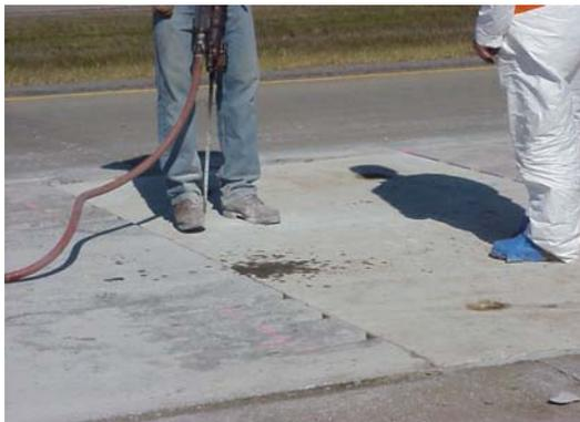
c) Drilling of injection portholes.
