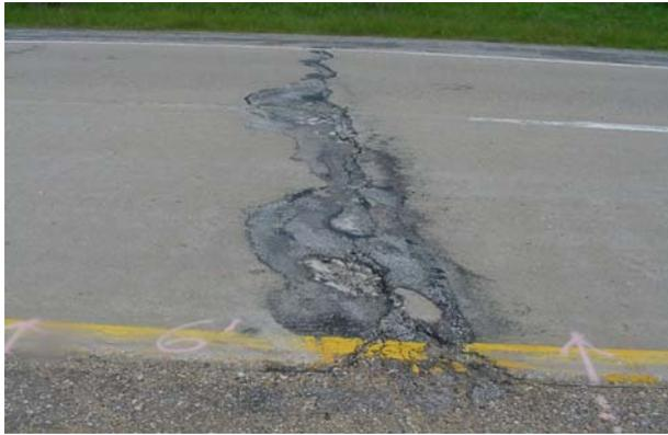
a) Deteriorated joint with cold patch with spalling.
