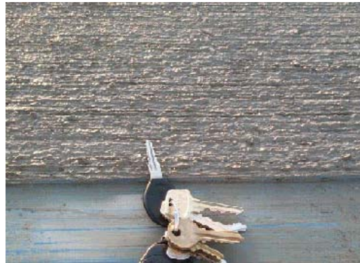
Figure 4.16 Creating surface textures by a carpet drag finish
