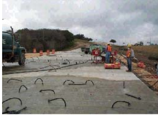
Figure 4.33 Grout the post tensioned conduits
