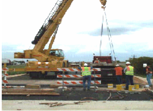
Figure 4.22 Transport panels to worksite
