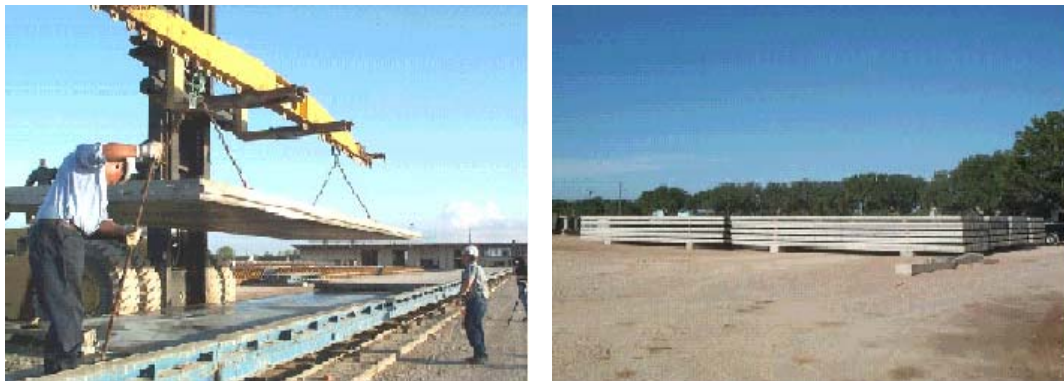
Figure 4.19. Move the finished panels to storage yard
