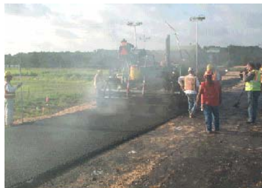
Figure 4.21 Place a 1"-2" thick asphalt leveling course on subbase
