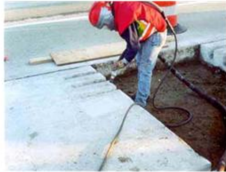
Figure 7.4 Cutting and Sandblasting of Dowel Slots (24)
