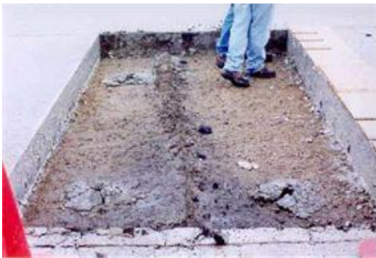
Figure 7.3 Base Preparation (24)
