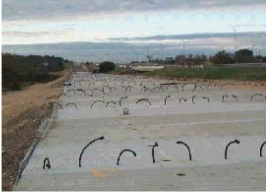
Figure 4.33 Grout the post tensioned conduits
