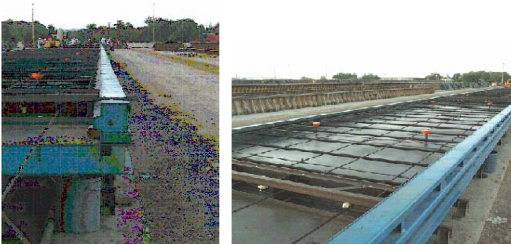
Figure 4.8 Looking down the side (left) and from the top (right) of the casting bed
