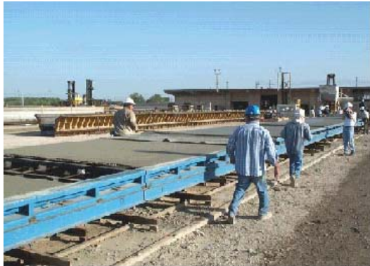
Figure 4.16 Creating surface textures by a carpet drag finish
