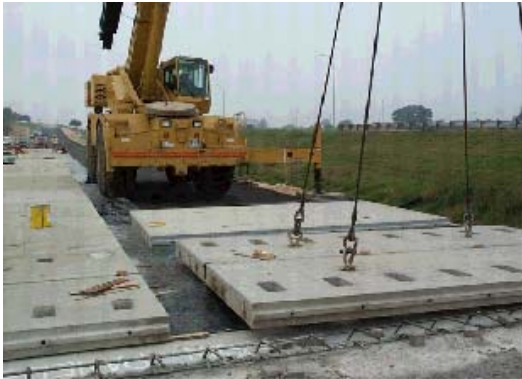
Figure 4.34 Assemble partial panels
