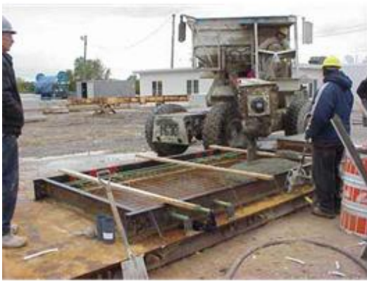
[c] Pouring Concrete
