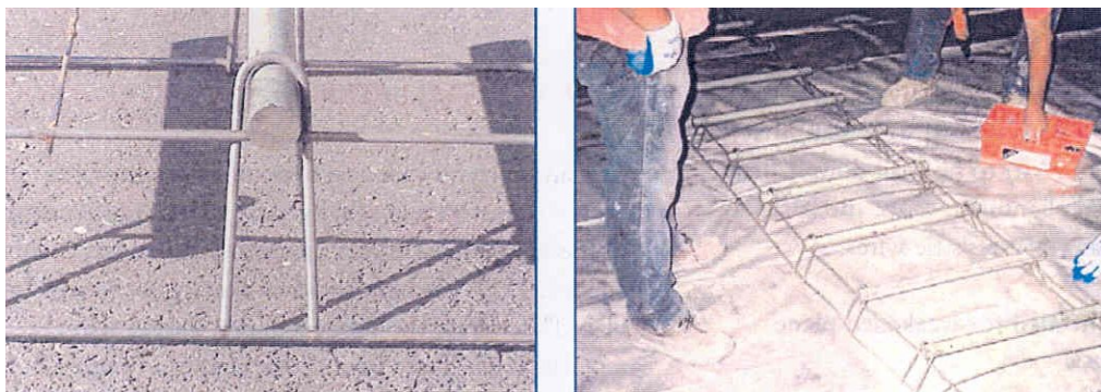
Figure 8.7 Type U Dowel Bar Basket (25)
