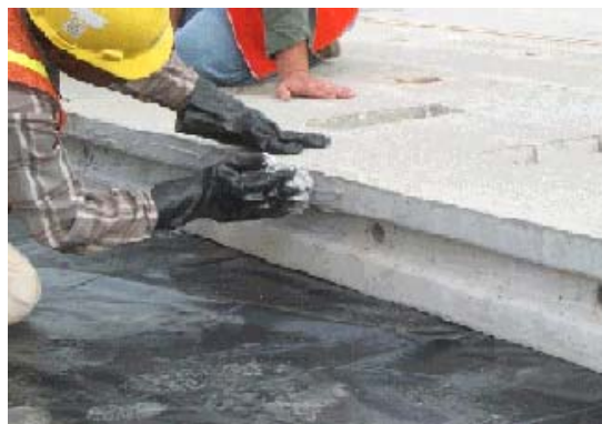
Figure 4.25 Place slow-setting epoxy
