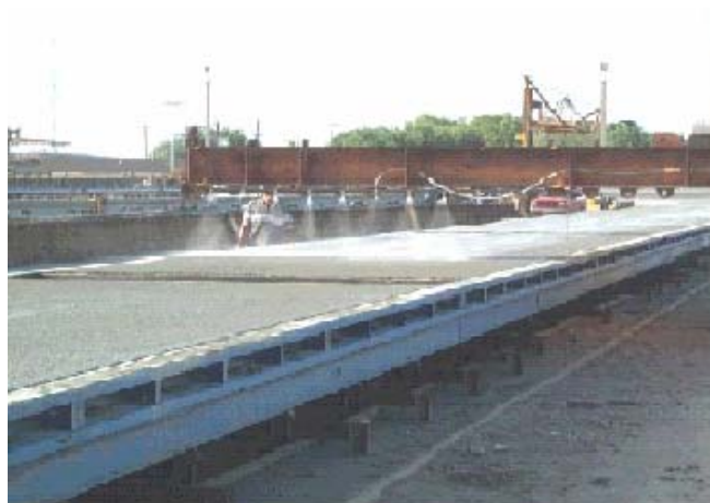
Figure 4.17 Double-coat of curing compound was applied
