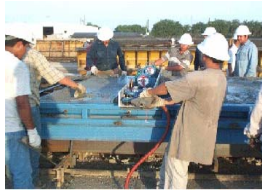
Figure 4.15. Leveling the surface of the concrete
