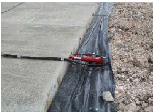
Figure 4.36 The post-tension is applied
