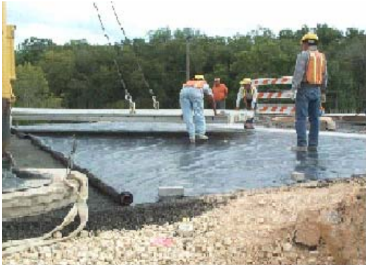
Figure 4.23 Place 1/8" polyethylene sheet on asphalt course
