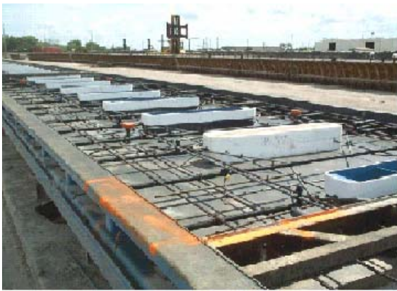
Figure 4.10. "Boxes/inserts" are placed for preparing the stressing pockets of central stressing panel mold
