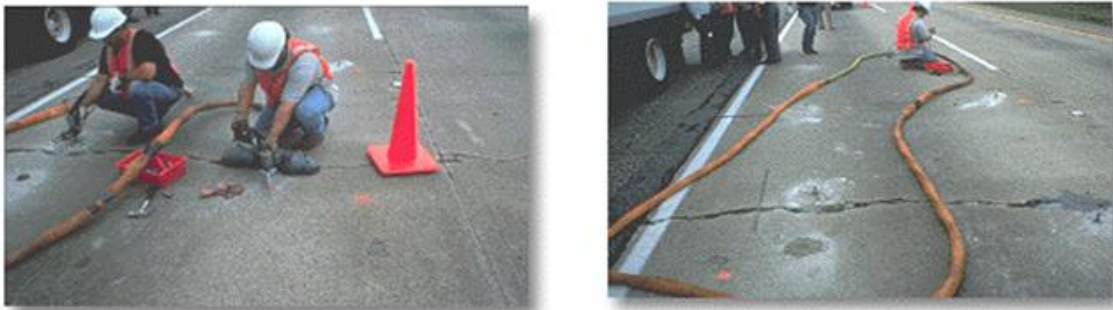
Figure 6.1 Uretek Method (21, 22)
