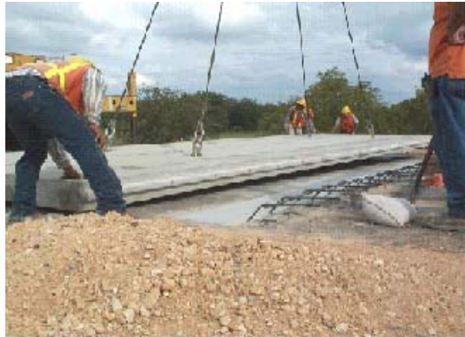
Figure 4.24 Place a full-width joint panel over the asphalt leveling course.
