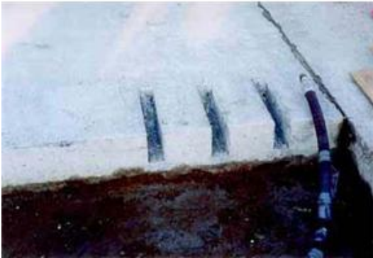
Figure 7.4 Cutting and Sandblasting of Dowel Slots (24)
