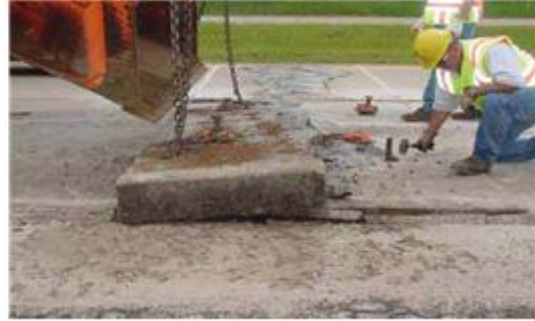
Figure 7.2 Lift Hook Installation and Slab Removal (24)
