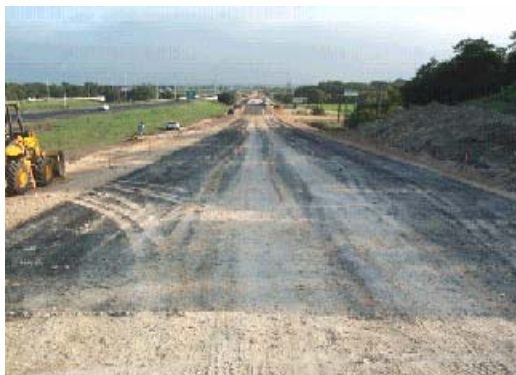
Figure 4.20 Preparing subbase
