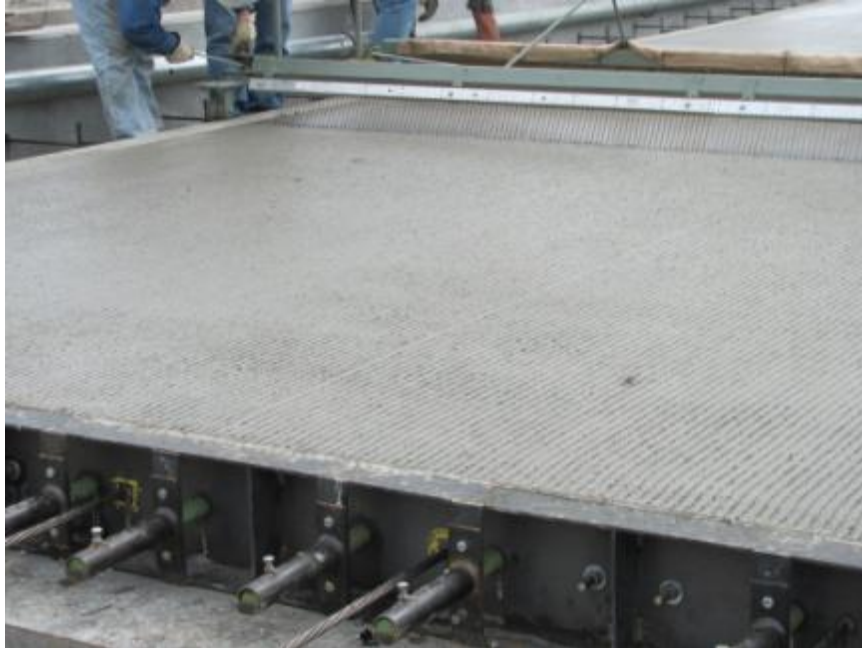
Figure 6 – Final Surface Finish
