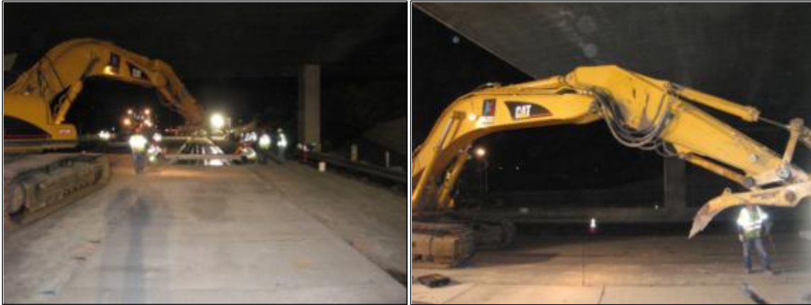
Figure 11 – PPCP installation under a structure (17' clearance)
