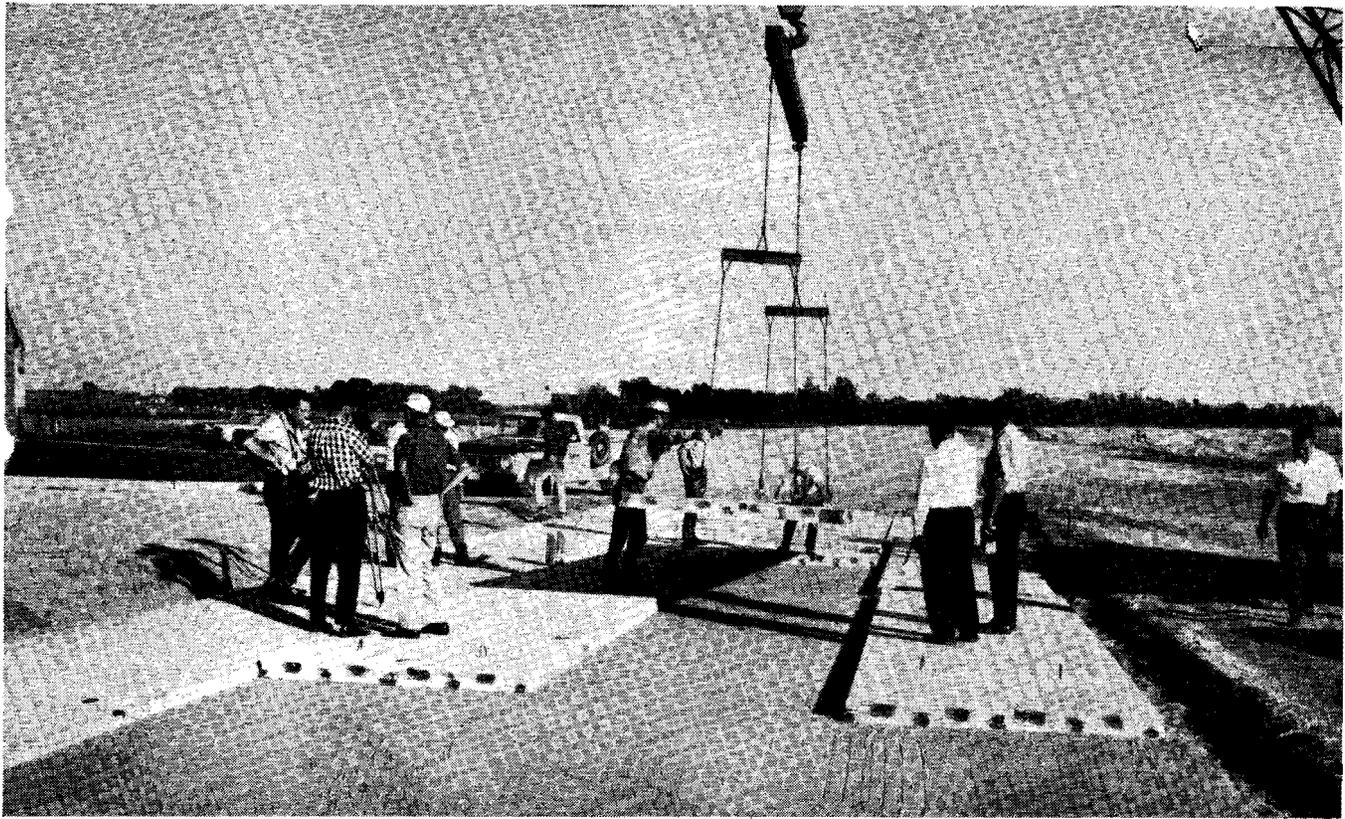
Placing a section of prefabricated highway.
