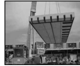
Jointed System - Ft. Miller SuperSlab™
