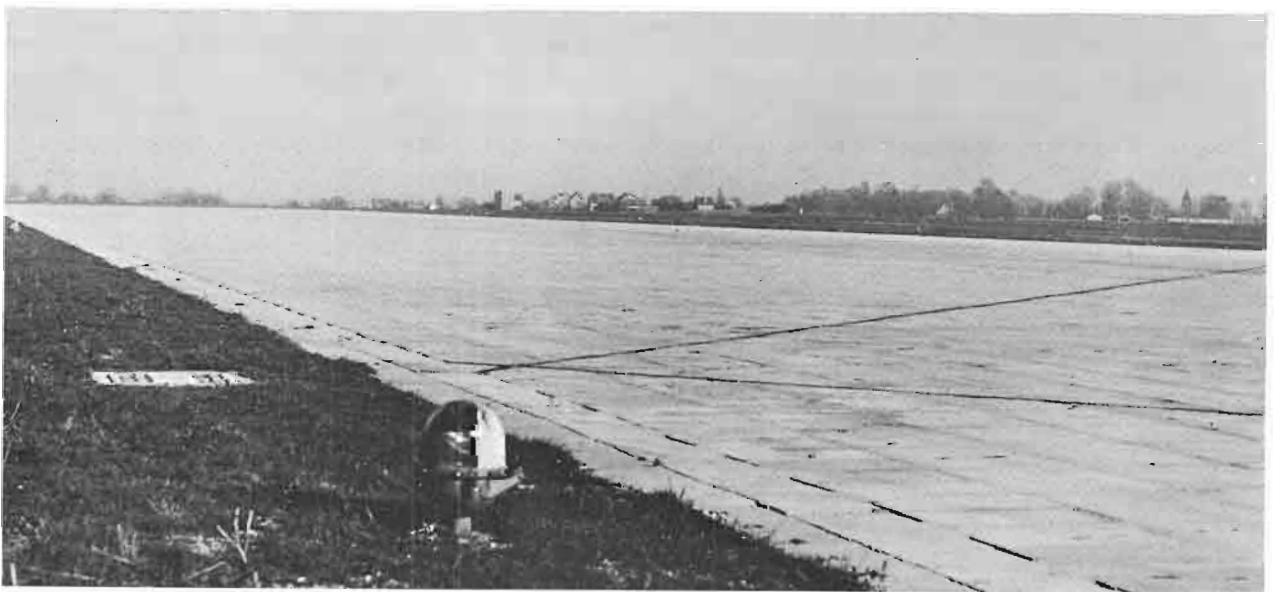
Figure A: Orly Airport. Prestressed concrete experimental length of runway, 1947.
